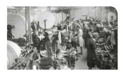
**1920s** — Production moved away from leather and towards woven transmission belting, laying the foundations for the development of heavyweight conveyor belting for coal mines that came in the 1950s.
